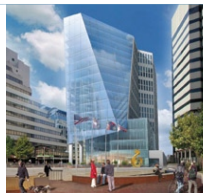
4 BETHESDA METRO CENTER The Meridian Group Bethesda, Maryland
