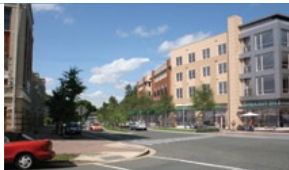
2201 NORTH PERSHING DRIVE Abbey Road Property Group; MacFarlane Partners Arlington, Virginia
